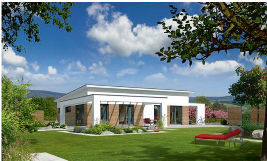
Fig. 9.7 Bungalow-type house with flat roof, tilted to sun direction (Courtesy: Holger Linke, Fingerhut Haus, Neunkhausen, Germany)
